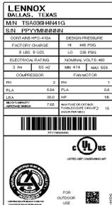
**Figure 54. Using HFC-410A Weigh In Method**
